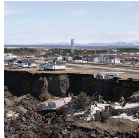
Figure 12.9 Heavy rains at the top of the cliffs and erosion at the bottom of the cliffs caused landslides in Daniel's Harbour on Newfoundland's west coast in 2006 and 2007.
