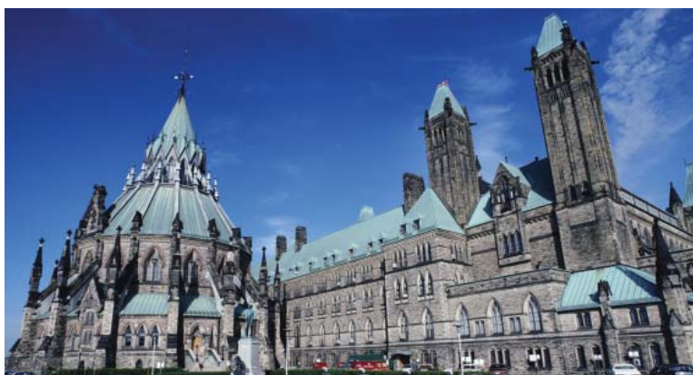
Figure 3.14 Corrosion has turned the roof of the Parliament Buildings in Ottawa from a red-brown to a blue-green colour.
