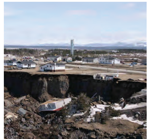
Figure 12.9 Heavy rains at the top of the cliffs and erosion at the bottom of the cliffs caused landslides in Daniel's Harbour on Newfoundland's west coast in 2006 and 2007.
