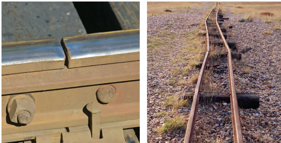
Figure 5.16 (A) Notice the space between each piece of iron track. The space is necessary so that, when the track expands in the heat, the rails will not push on each other and cause bending. (B) This is what happens if not enough space was left between the pieces of track.
