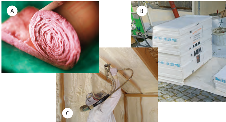
Figure 6.23 (A) Insulation often comes in rolls of a soft material called batt that is placed between the wooden beams in a wall. (B) Solid foam sheets of insulation are used for some situations. (C) Some builders prefer a spray foam that is applied directly to the structure of the building.
