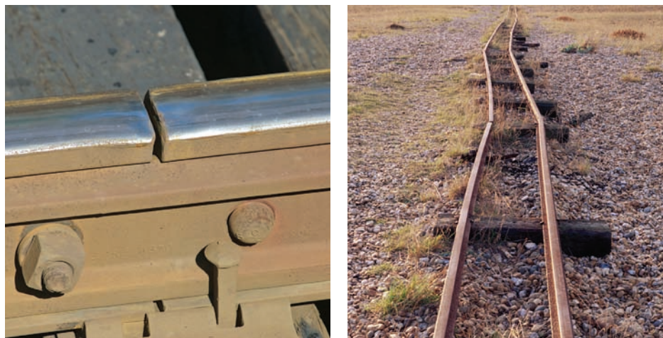
Figure 5.16 (A) Notice the space between each piece of iron track. The space is necessary so that, when the track expands in the heat, the rails will not push on each other and cause bending. (B) This is what happens if not enough space was left between the pieces of track.
