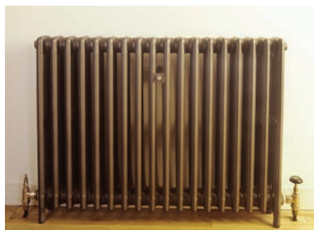
Figure 6.18 Baseboard heaters and radiators heat air by conduction with the air particles that come in contact with the metal surface. The hot air distributes the heat throughout the room by convection.
