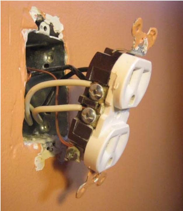
Figure 9.16 Electrons flow into and out of a device through the two slots in a wall outlet. The round hole in a wall outlet is connected to a ground wire like the copper wire shown in this photo.
