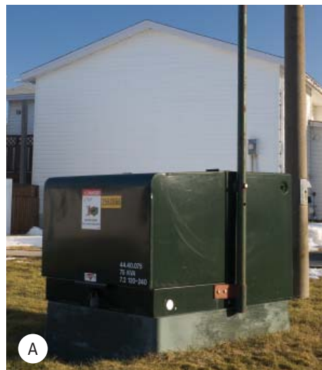
Figure 9.36 Transformers step down the voltage before a line is connected to the meter at your home. Transformers are located either inside a green box (A), or on the power pole (B).
