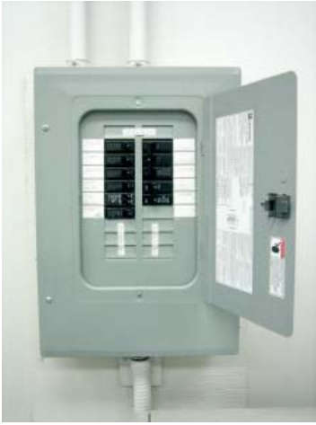
Figure 9.14 The service panel, often found in the basement of a house, is the junction point from which a number of parallel circuits originate. Each circuit is protected by its own circuit breaker.
