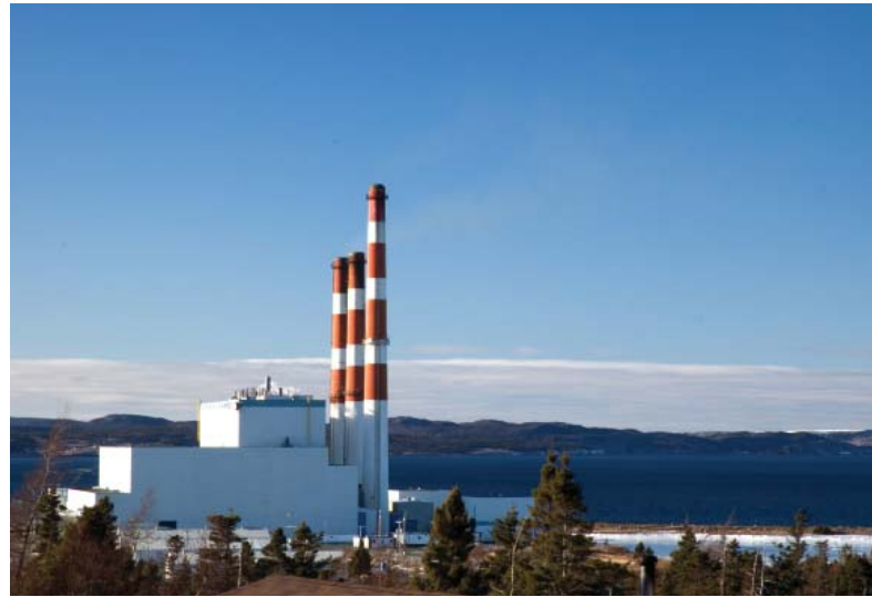
Figure 9.39 The Holyrood Generating Station burns heavy fuel oil, a non-renewable energy source.
