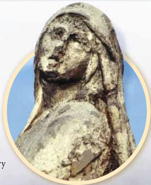
This photo shows a statue after it has been exposed to acid deposition.
