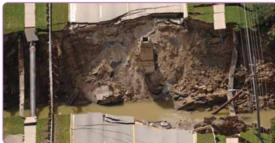
Figure 7.26 When this street collapsed in Toronto in 2005, it damaged two high-pressure gas pipes, a drinking-water pipe, and telephone, hydro, and cable service lines that were buried beneath the road.
