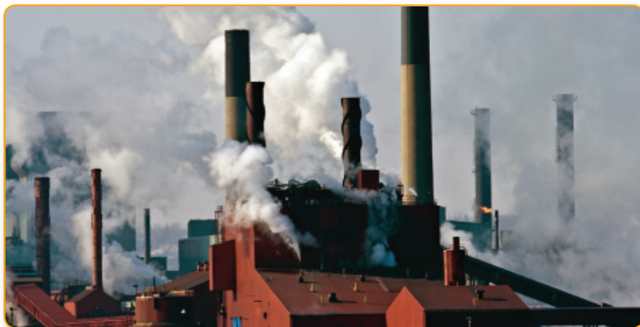
Figure 10.19 Most of the “smoke” you see coming from the smokestacks on this steel plant in Hamilton, Ontario, is condensing steam. However, the emissions also contain harmful substances that an electrostatic precipitator can remove.
