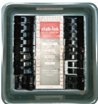
► Figure 4.33 Every switch in a circuit panel controls one parallel circuit. Circuit breakers are always located beside the source. When they break the circuit, no current flows to any of the pathways. The circuit breaker in the diagram will open the circuit when the current goes above 15 A.
