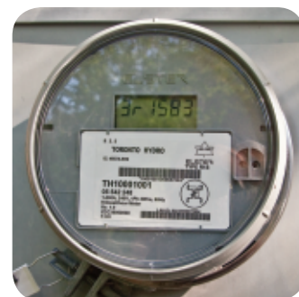
▲ Figure 4.39 The new smart meters measure energy use each hour. The meters encourage “smart” behaviour on the part of Ontarians by giving us the means to think about how and when we use electrical energy.
