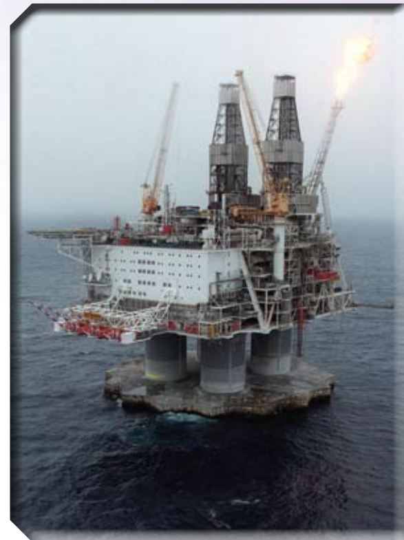
Figure 15-9 In 1999, this Hibernia oil platform extracted oil about 315 kilometres southeast of St. John's, Newfoundland. The provincial and federal governments disagreed over sharing royalties from the oil industry. How might this disagreement affect national unity?
