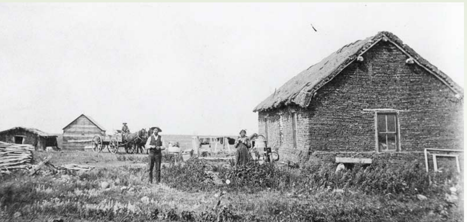
Figure 13-10 This photograph of a sod house was taken near Viking, Alberta, in the early 20th century. The first house of many Prairie homesteaders was either built completely of sod, like the one pictured, or had a sod roof.
