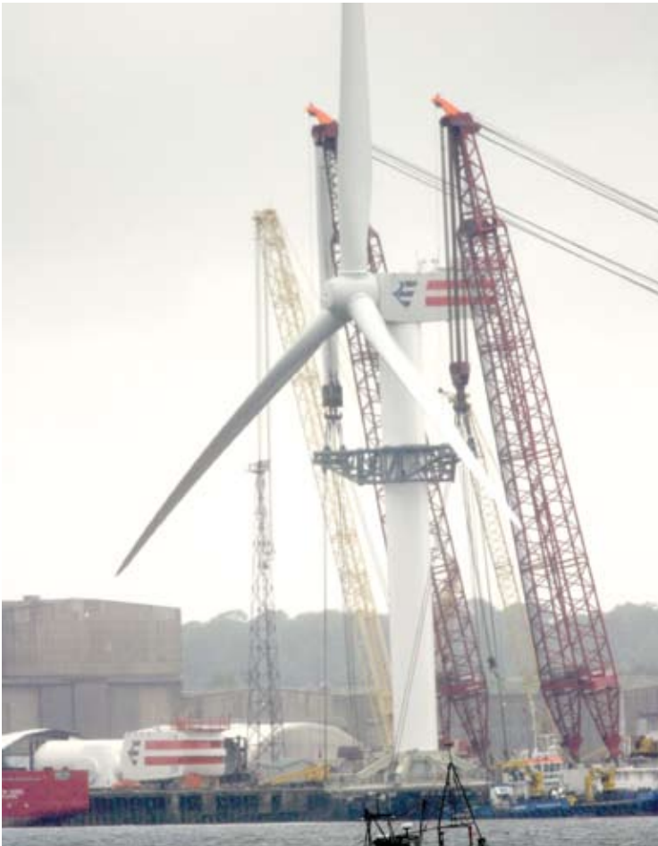
Figure 10-19 In August 2006, the first of two huge wind turbines developed by Talisman Energy and a consortium of other companies was transported to a location in the North Sea. The blades of the turbine are 63 metres long, and the structures will tower 170 metres above sea level.
