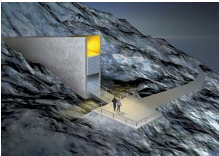
Figure 12-20 The Svalbard Global Seed Vault will be built deep inside a mountain. Scientists believe that the thick rock and permafrost will ensure that millions of seed samples from around the world will remain frozen. This drawing shows what the entrance to the vault was to look like.
